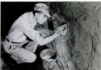
Scrub damp-proofing into wall with stiff brush.
